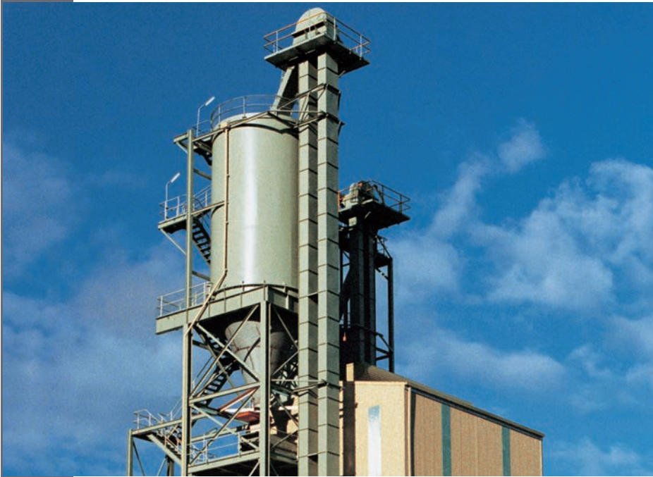
Silo feeding by means of high-performance bucket elevator with central chain.
