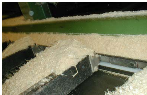
Wood chips conveyor in sawing line
