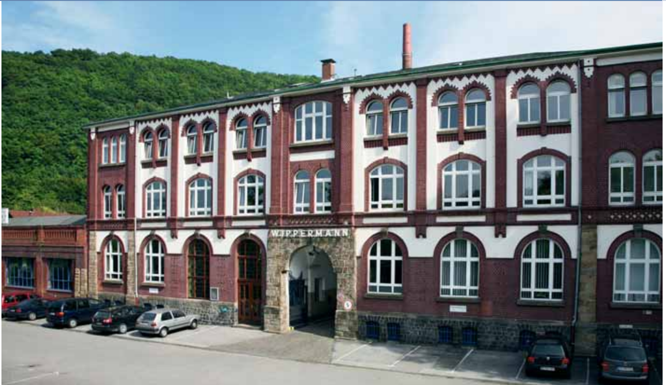
Wippermann administration building
