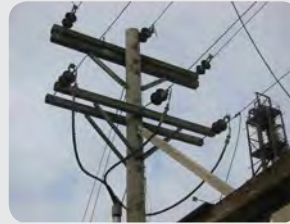
Distribution line faults
